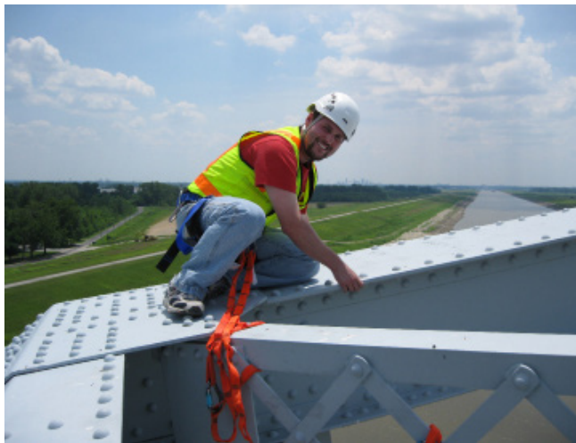
Adam inspecting the top of the Old Chain of Rocks Canal Bridge
