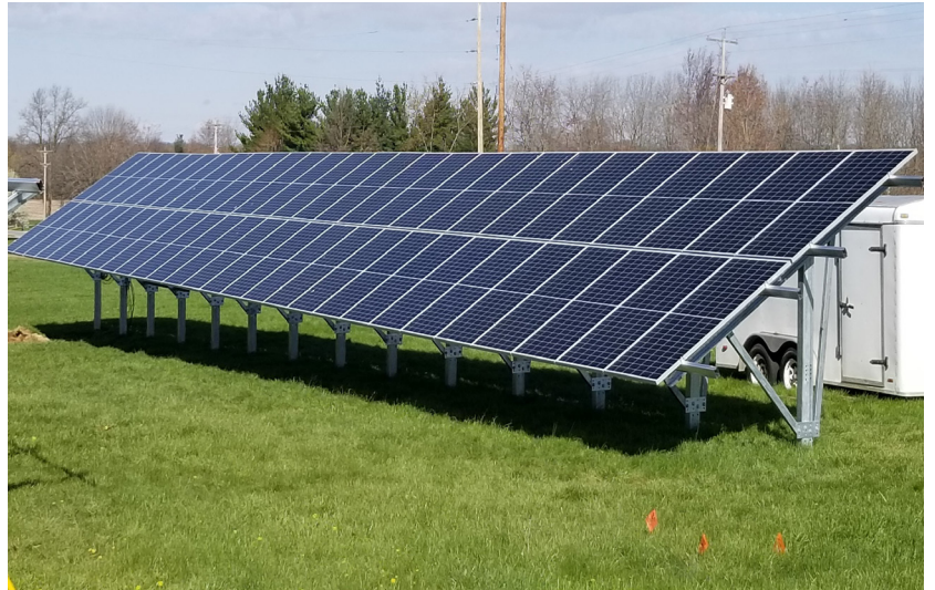
Installation of the first section of solar panels
