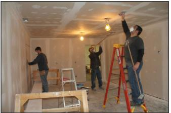
Students enrolled in the Construction Technology Program continue to work at the Wayne County Well Surveys. Most recently they have been installing drywall, mudding the seams, and sanding to a smooth finish. Once the drywall is comepleted, students will install a ceramic tile floor, and add kitchen cabinets and counter tops.
