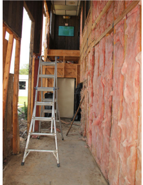
Due to termite damage, the west wall and stairway are being removed and then will be rebuilt.
