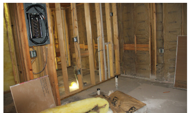
Bottom right: Plumbing and electrical boxes are set in the room that will house the ice machine and utility room.
