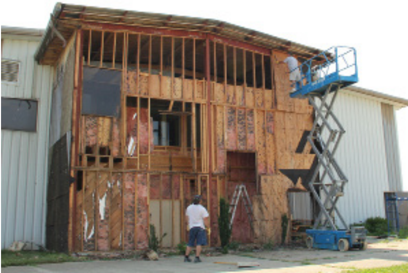
Due to termite damage, the west wall and stairway are being removed and then will be rebuilt.
