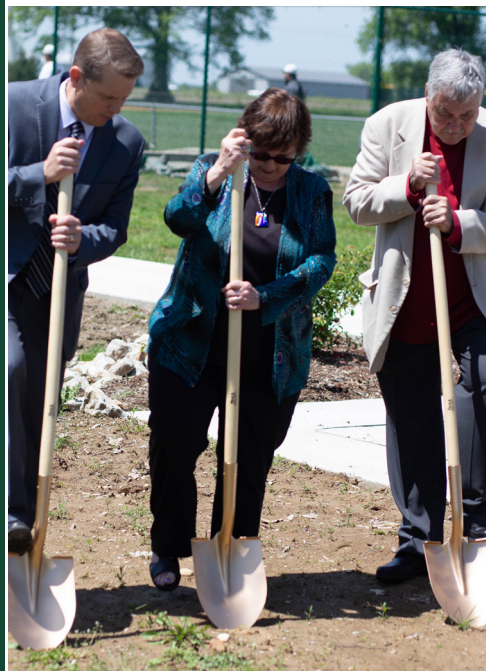
LTC President Ryan Gower, Foundation President Sheila Mikeworth and Foundation Executive Director Rod Harmon break ground.
